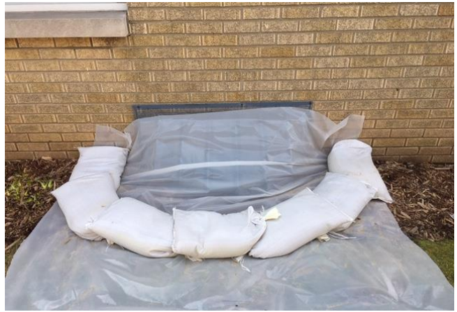
2. Lay a sheet of plastic down and place one row of sandbags around window leaving at least six inches (6") on each side and one foot (1') in front. Overlap bags slightly.
