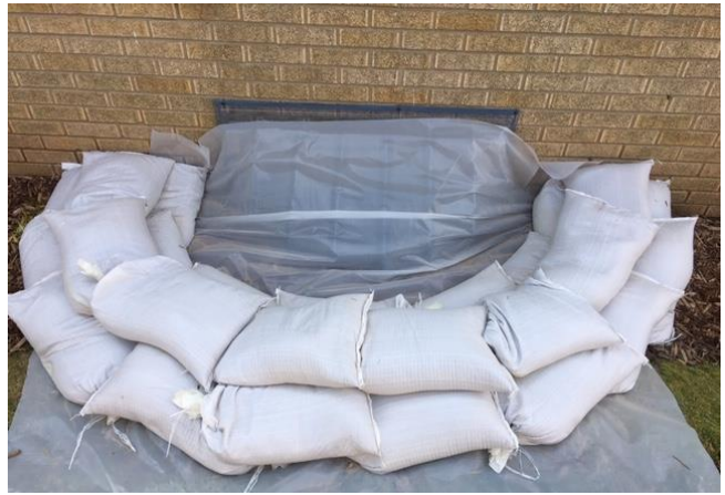
4. Place a third row of sandbags on top of the first two (2) rows, overlapping two (2) base rows and each sandbag as you go.
