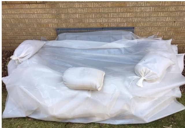
5. Pull plastic up and over sandbag wall, placing a few bags on top to hold plastic in place.
