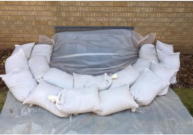
3. Place a second row of sandbags next to the first row using the same method.
