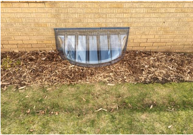
1. Picture of the window before.
