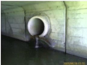
**Dry Weather Flow** is noted when it has not rained for at least 72 hours and the storm drain has flow or the drain shows signs of intermittent flow (staining and odor).
