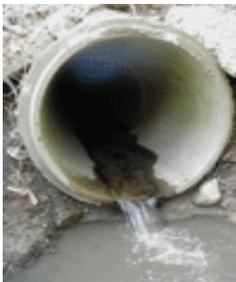
**Sanitary Sewage** may be present if there is black staining inside the drainage pipe; visible evidence of sanitary waste, such as toilet paper; or opaque or gray water. Sewage may originate from septic tank overflow pipes or improperly dumped travel trailer waste.
